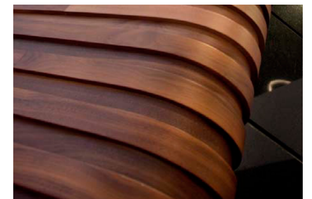
Hotel lobby – veneered wall detail
